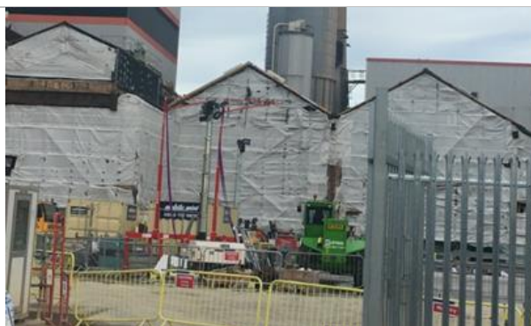
Photo 8. B9 under demolition/refurbishment
